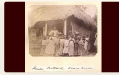
House in Bathurst, Sierra Leone, c. 1870 NA, CO 1069/88 Download No additional info
