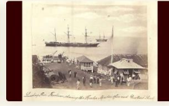
Landing Pier, Freetown, c. 1870 NA, CO 1069/88 Download No additional info
